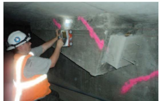
Using data from high frequency GPR technicians mark duct location on the surface of the concrete for further sonic/ultrasonic testing.
